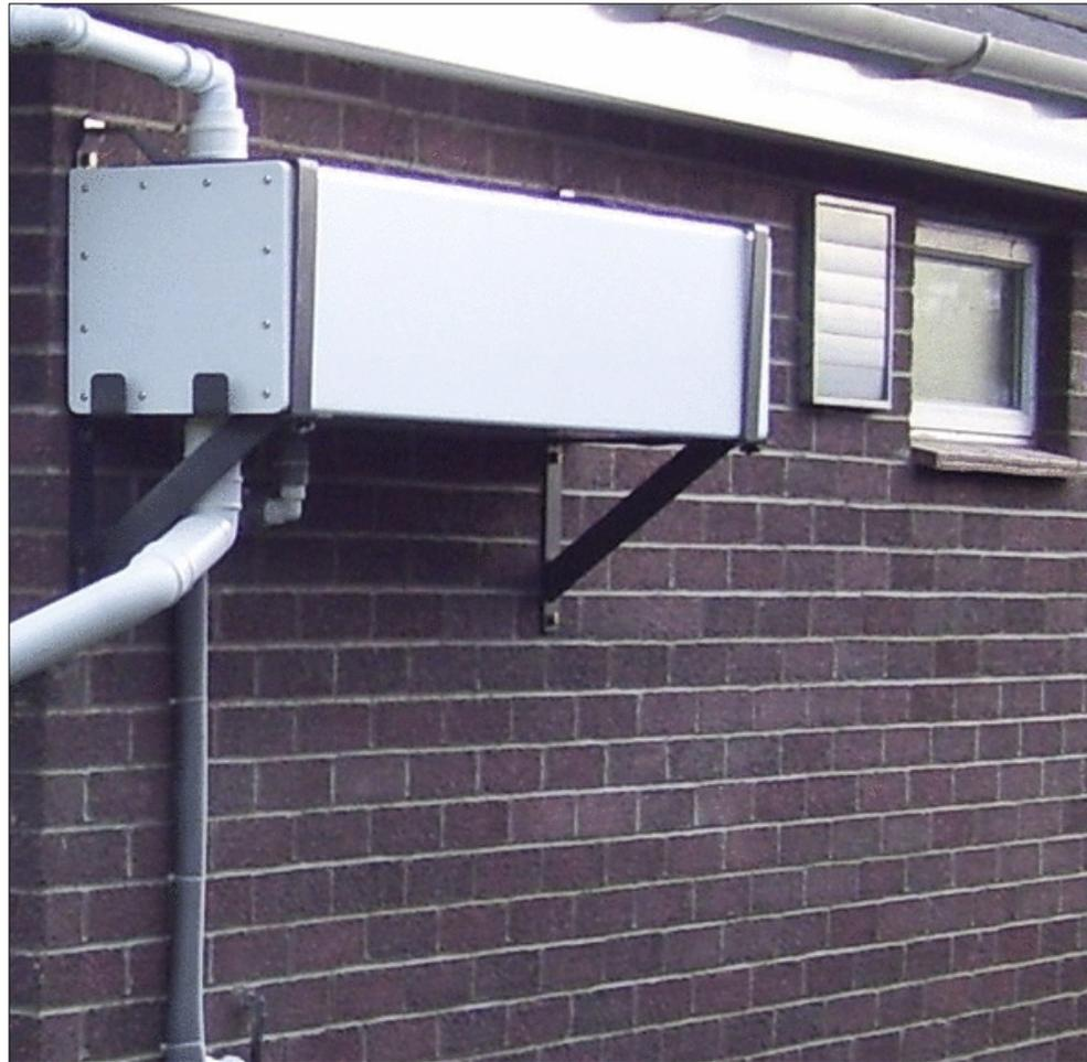
**Dwr Cymru/Welsh Water**, consultants **MWH** and manufacturer **Aqualogic** are working to produce affordable wall-mounted rainwater harvesting systems
