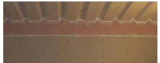
Typical partition head detail found in schools, undergoing tests in the chamber
