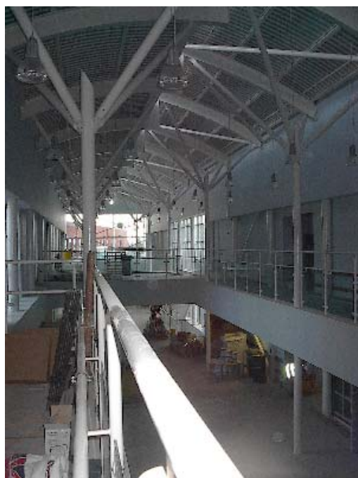
The main atrium at St James School, Exeter
