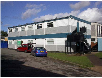
Examples of relocatable classrooms which were tested for BB93 compliance. Reverberation times were short due to low ceilings, and decent levels of acoustic separation were achieved between classrooms where there was an intervening space (e.g. lobby)
